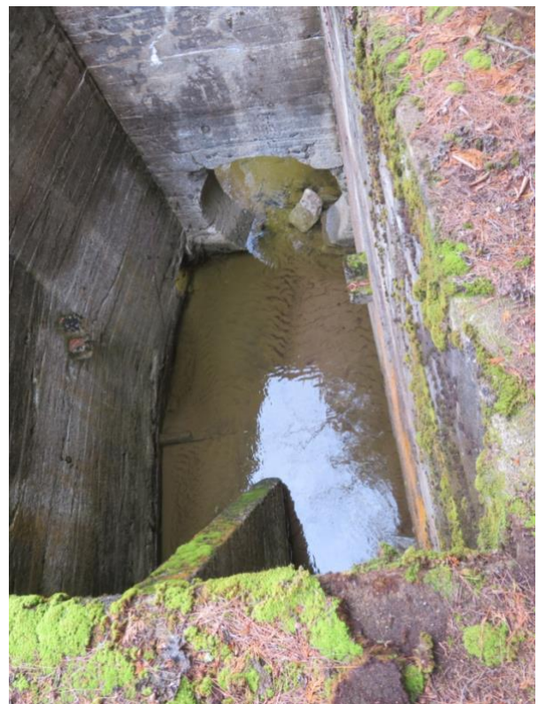
Inside view of the intake structure showing the exit hole for the penstock (referred to as a "flume" in early newspaper accountry).
