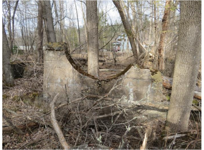
Concrete support for the penstock. Located just downhill of the trench, this is likely where the penstock entered the saw mill/ power plant. The Mountain Health Center is visible through the trees.
