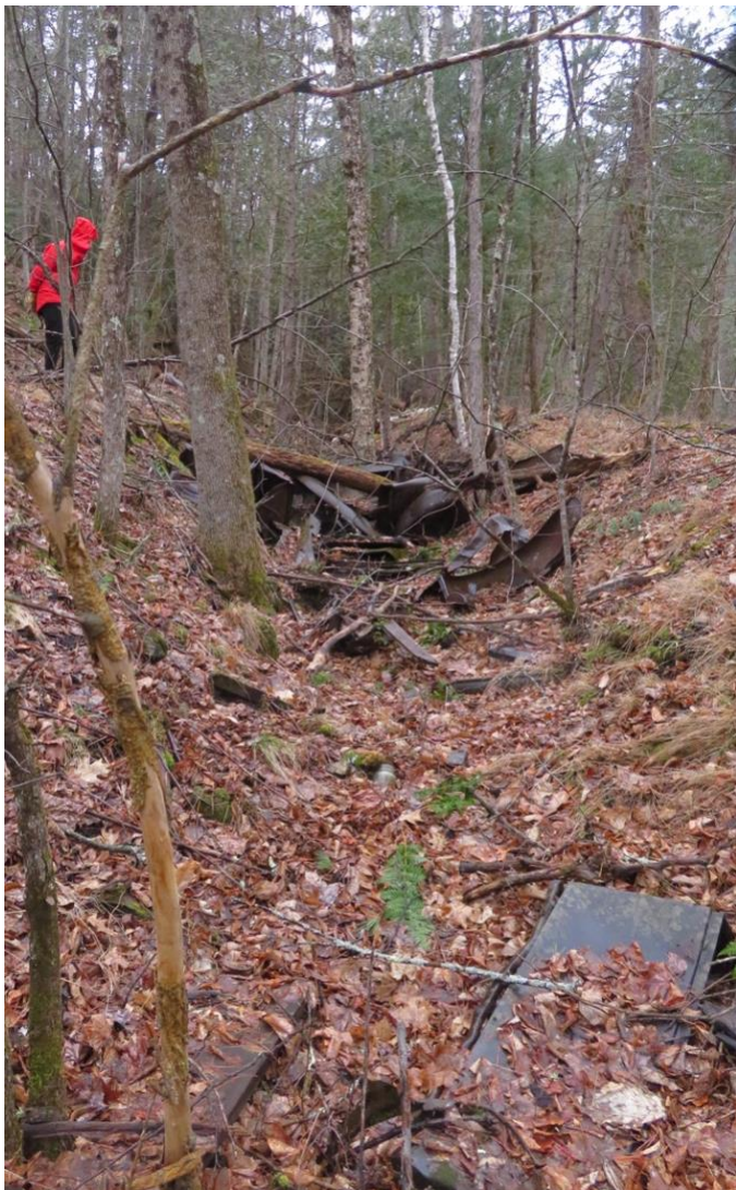
Trench that held the penstock that brought the water from the intake to the sawmill/power plant. The metal debris is of an old vehicle, not the original penstock, or flume..
